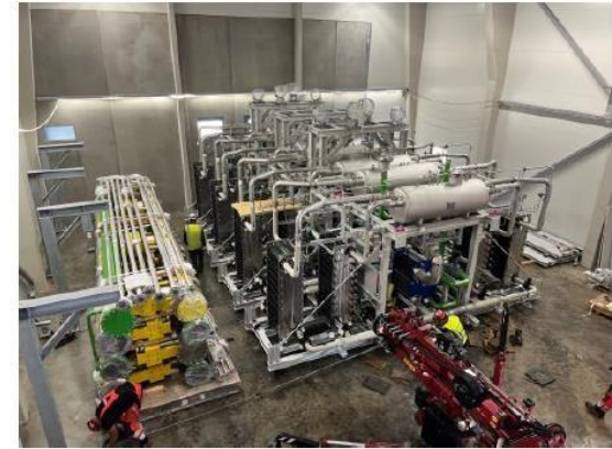
2nd electrolyzer (out of 3)
