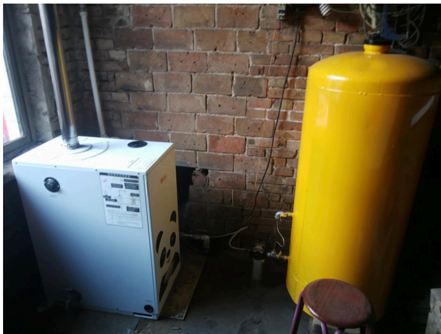
Pic 28: Retrofitted methanol fuel boiler in Jinzhong city
