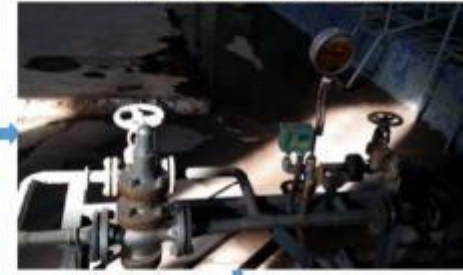
Fuel Metering and Mixing
