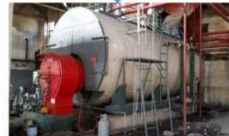
Methanol Boiler
