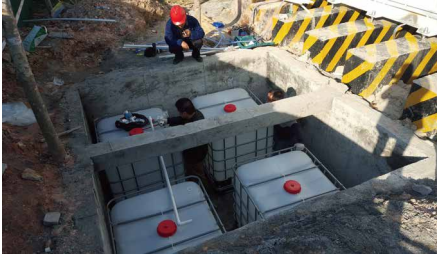
Two 2kW aqueous hydrogen generators in parallel for Guangzhou Zengcheng Xiangshan base station
