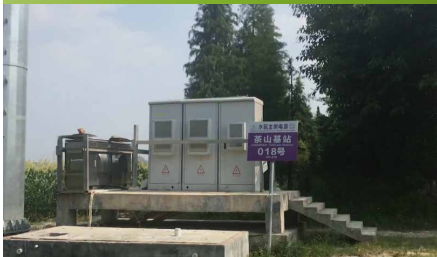
Two 2kW aqueous hydrogen Generators in parallel for Dongguan Chashan telecom Base station
