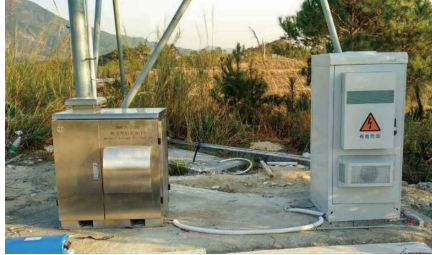
One 2kW aqueous hydrogen generator for Huizhou Huidong base station
