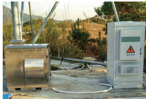
Aqueous hydrogen generators as backup power supply
