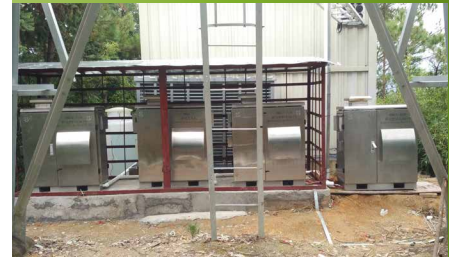
Four 2.5kW aqueous hydrogen generators in parallel for Guangzhou Conghua Huang gutian base station
