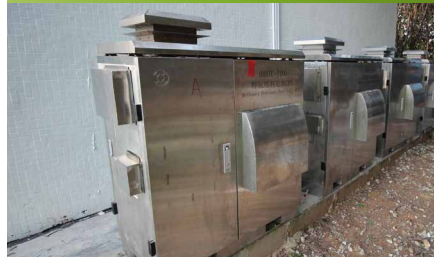
Four 2.5kW aqueous hydrogen generators in parallel for Guangzhou Zengcheng Nan xiangshan base station,
