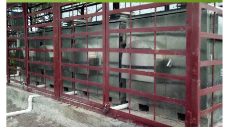
Four 2.5kW aqueous hydrogen generators in parallel for Guangzhou Conghua Shang Huanggutian Tian base station
