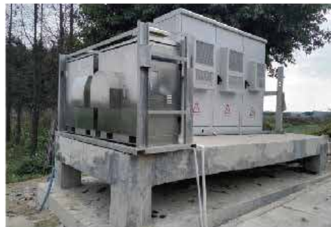
Aqueous hydrogen generators provide the long-term electricity
