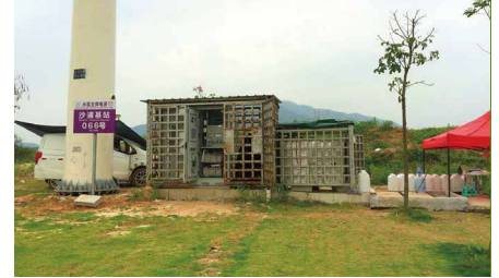
Two 2kW aqueous hydrogen generators in parallel for Guangzhou Zengcheng Shapu base station
