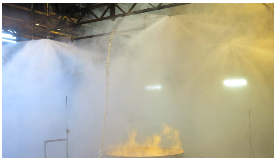
Figure 9. Activated Ultra Fog water-mist system providing nominally 1.5 l/m 2 /min.
