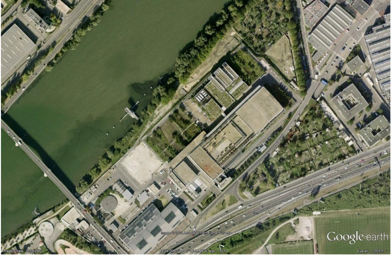
Figure 4-12. Seine-Centre WWTP. Source: Google Earth. Date of image: 10/20/2007
