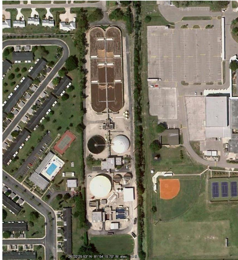
Figure 4-10. Fiesta Village Advanced WWTP. Source: Google Earth. Date of image: 04/01/2010
