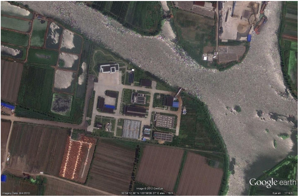
Figure 4-13. WWTP in Jiashan City, China. Source: Google Earth. Date of image: 08/04/2010
