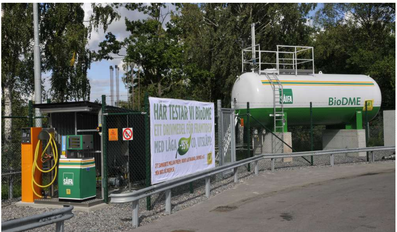
Figure 18. Bio-DME filling station in Sweden in 2011
