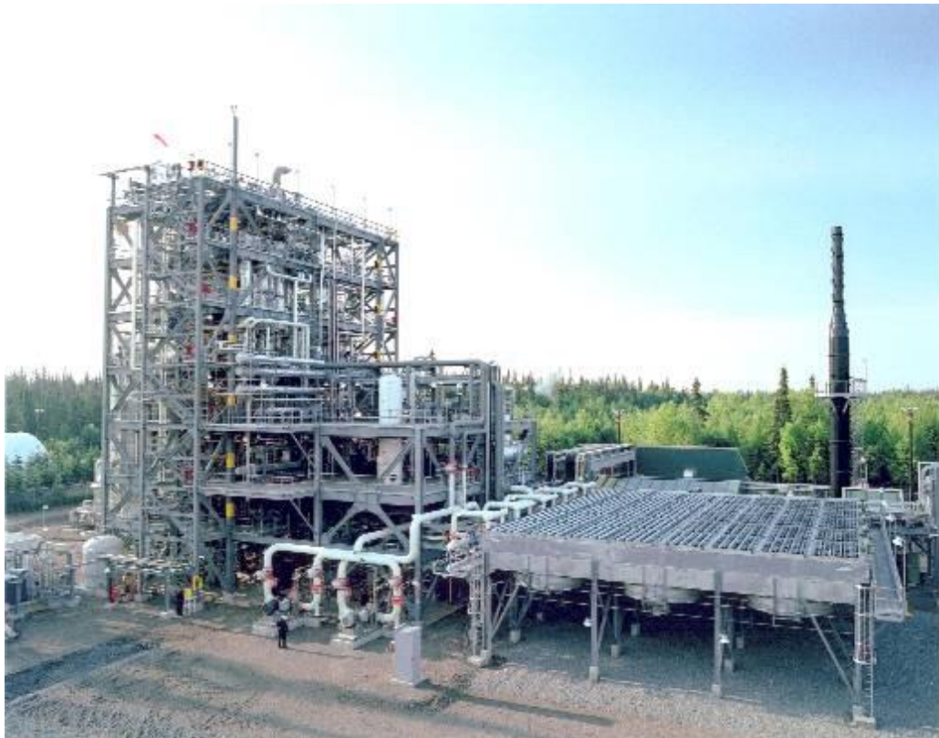
Figure 1 - DAVY compact reforming installed on the Nikiski demonstration plant.
