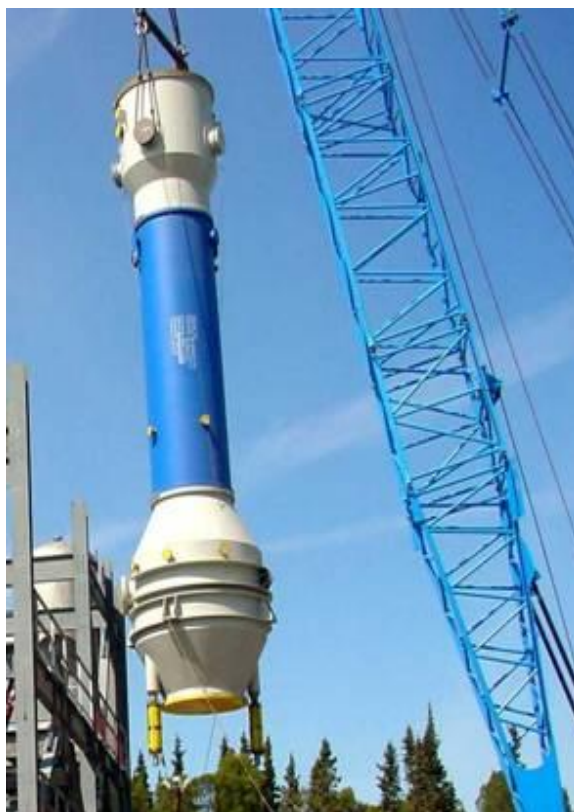
Figure 2 - Nikiski Compact Reformer module
