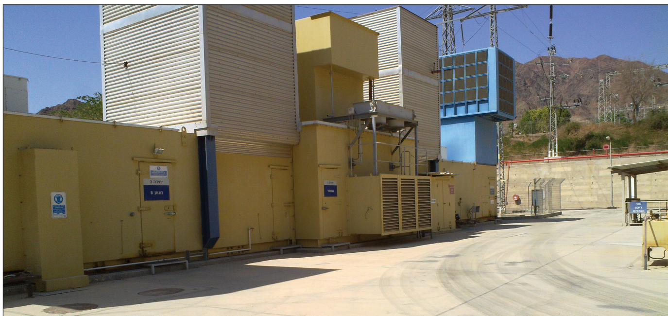
Figure 1. The Eilat generating plant. The gas turbines were converted to use methanol at the end of 2013.
