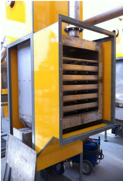
JM tar reforming catalyst installed in Ecorel 1MW el biomass CHP plant
