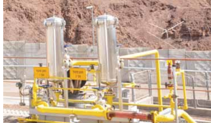
Methanol filters in the Eilat GT site
