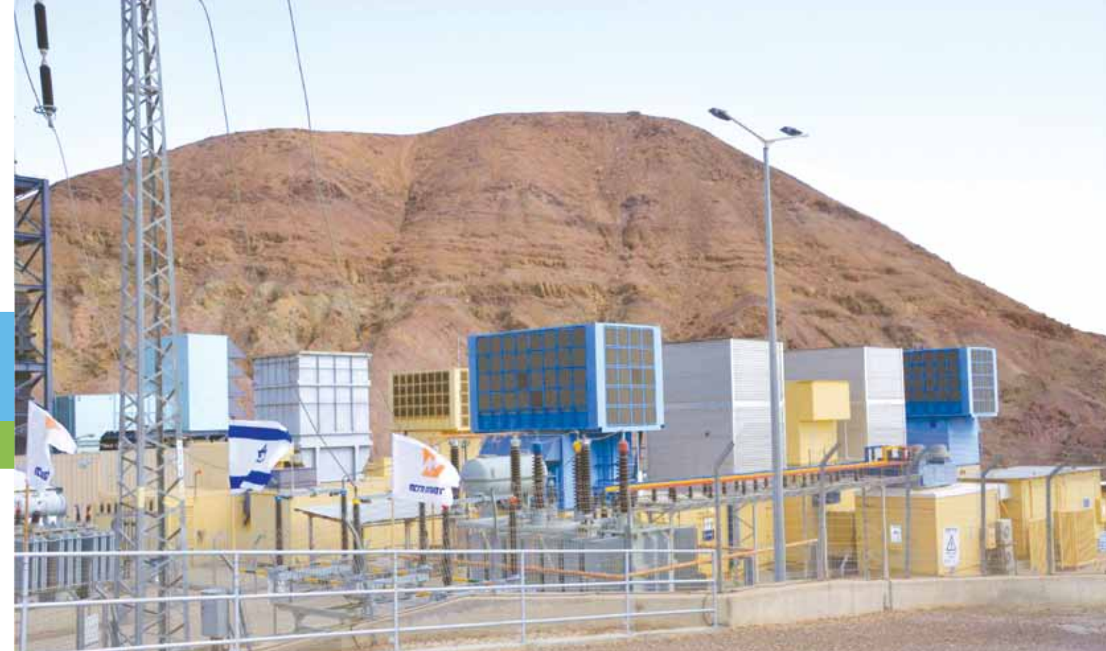
Overview of the Eilat GT site converted to methanol
