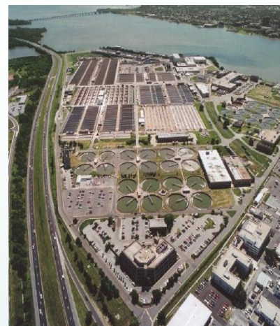
Blue Plains Wastewater Treatment Facility
