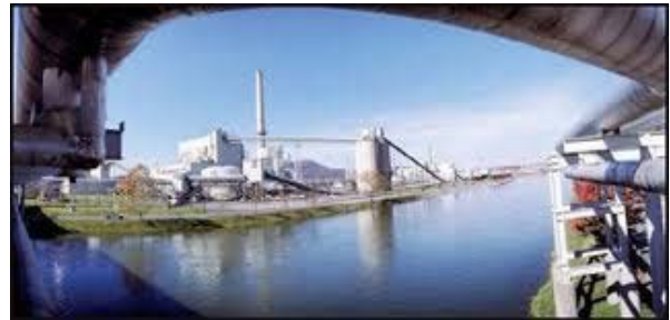
Kingsport, TN Methanol Facility.
